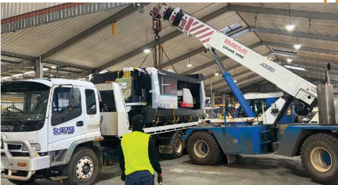
A crane lifts the new Omada Laser into its spot on the factory floor.
