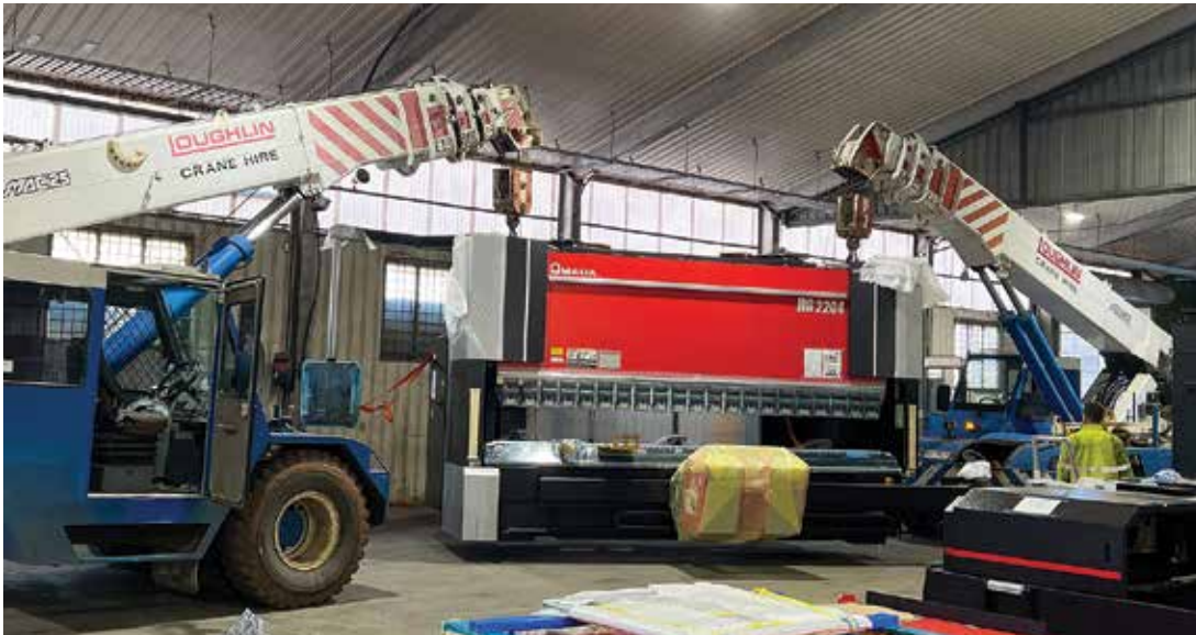
Two cranes lift the new press brake into place in the TUFF factory.
